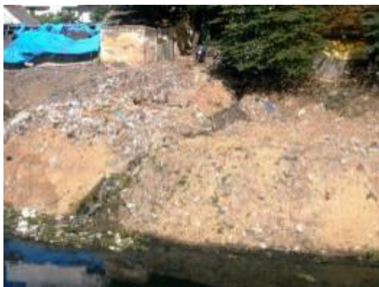
Picture 1. Raw sewage flow to the river in Metha Nagar
