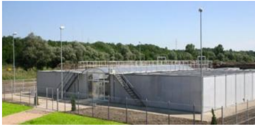
Picture 4. STP built with modules
